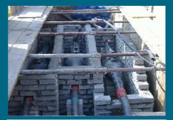
The 400 kV cables may be delivered in lengths of 800 to 900 meters, lower voltage cables may be longer.
